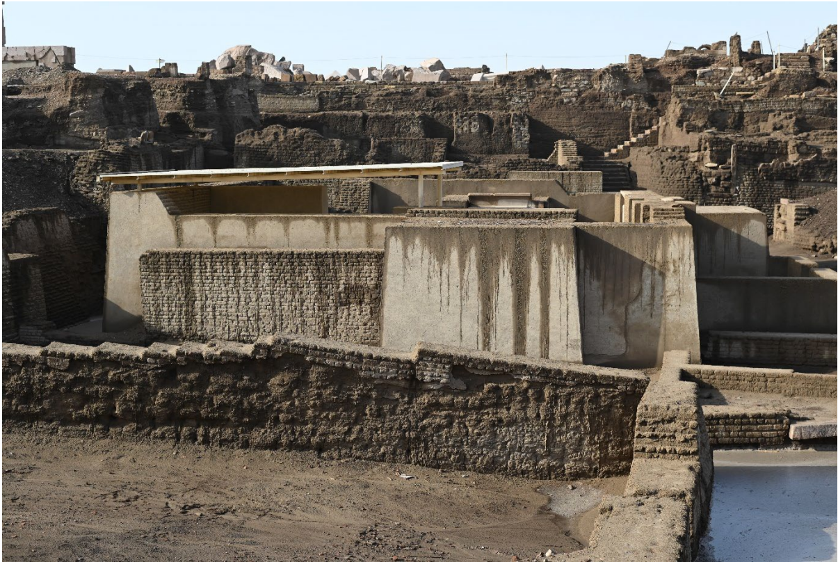
Fig. 14: Erosion of mud-brick masonry and plaster at the Sanctuary of Heqa-Ib, looking south (photo: M. Sählhof, © DAI).
