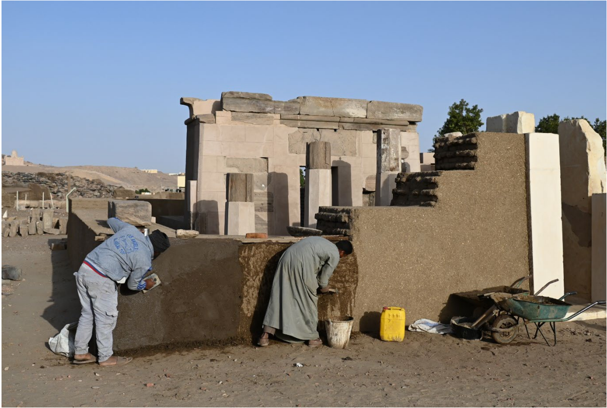
Fig. 17: The 11 th Dynasty Satet Temple (Mentuhotep II); Repairing of the mud plaster surface: the old, eroded surface (right), moistening and roughening (middle), and finally re-plastering (left), looking west (photo: M. Sählhof, © DAI).
