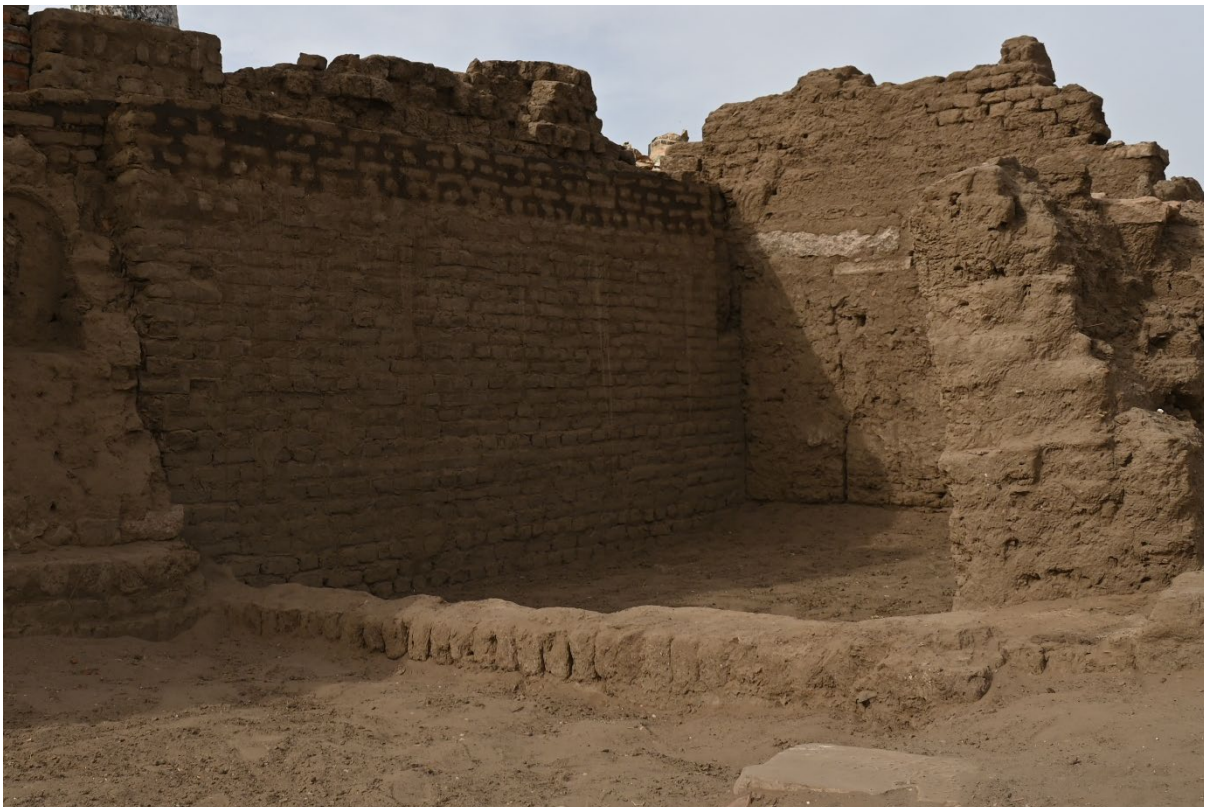
Fig. 15: At House M14, the western wall is supported with a facing shell, looking north-west (photo: O. Kassab, © DAI).
