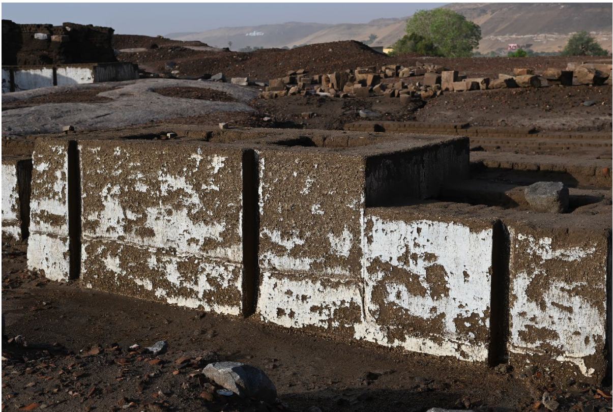
Fig. 13: Erosion of mud-plastered surfaces exposed to rainfall on the reconstructed Old Kingdom Mastabas, looking south (photo: M. Sählhof, © DAI).
